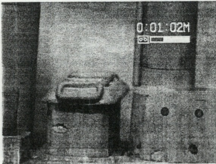
Hole in lower right corner of deckhouse was from funs of USS Houston.
