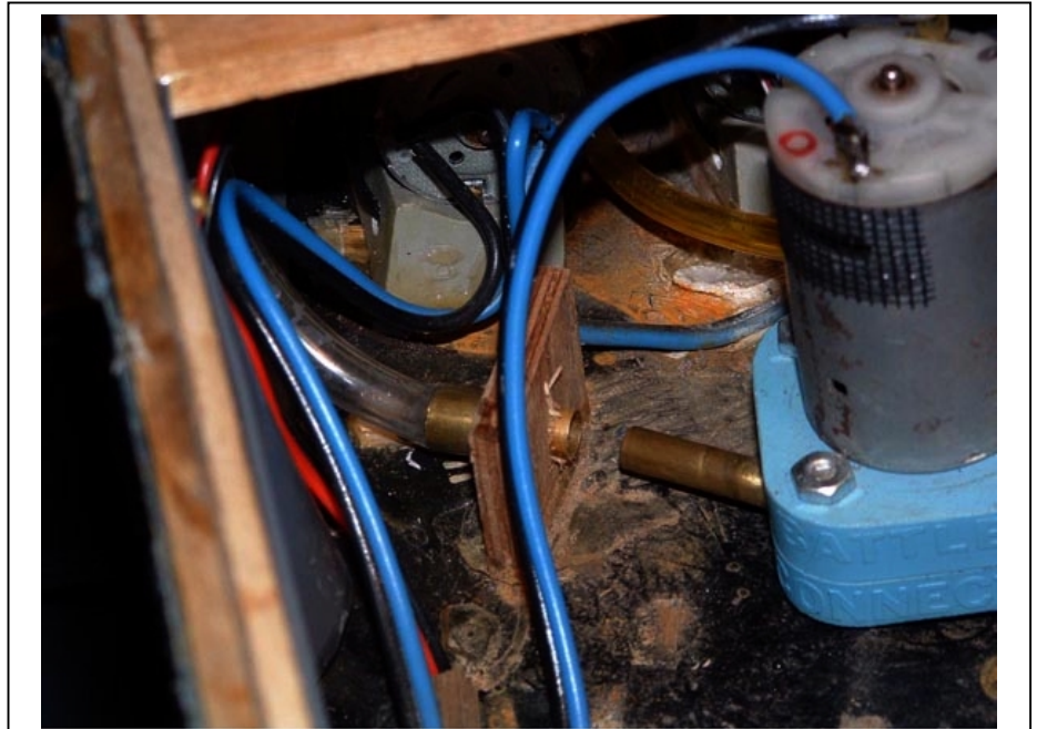
The new plug and spray system.
